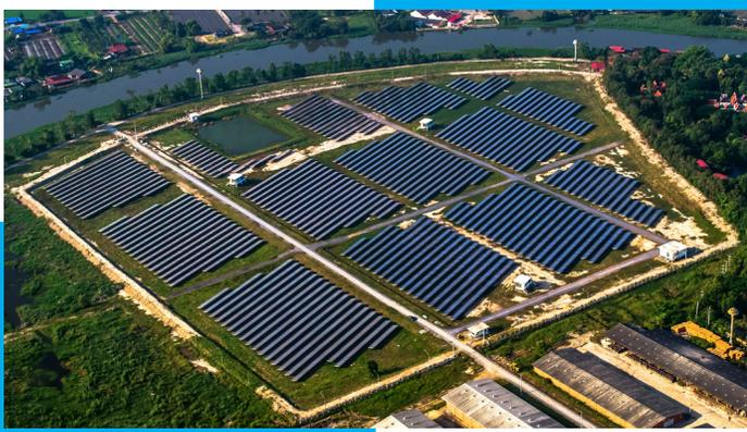
PV system production is limited by the output of the inverter that converts the DC power from the modules to AC power suitable for use by the grid. Typical system design dictates that the nameplate capacity of the modules (DC) should exceed the nameplate capacity of the inverters (AC output) by at least 20%, and often as much as 40%. The array is constructed larger on the DC side to compensate for times when irradiance (available sun energy) is reduced due to poor weather or time of year.
